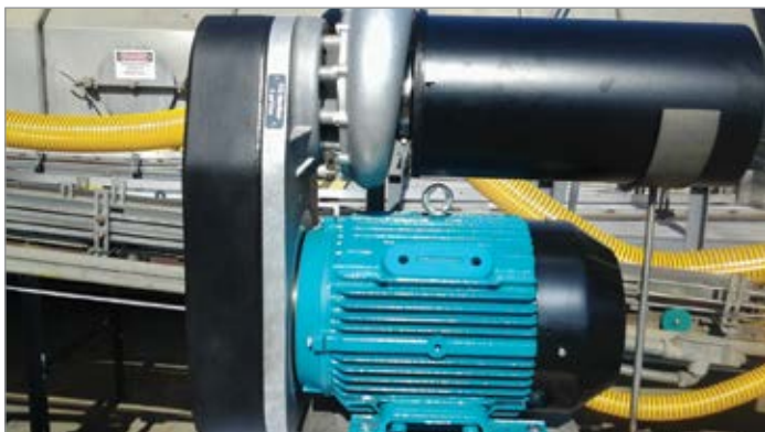
Image 1: Sample installation of the Vortron Z40e centrifugal blower
