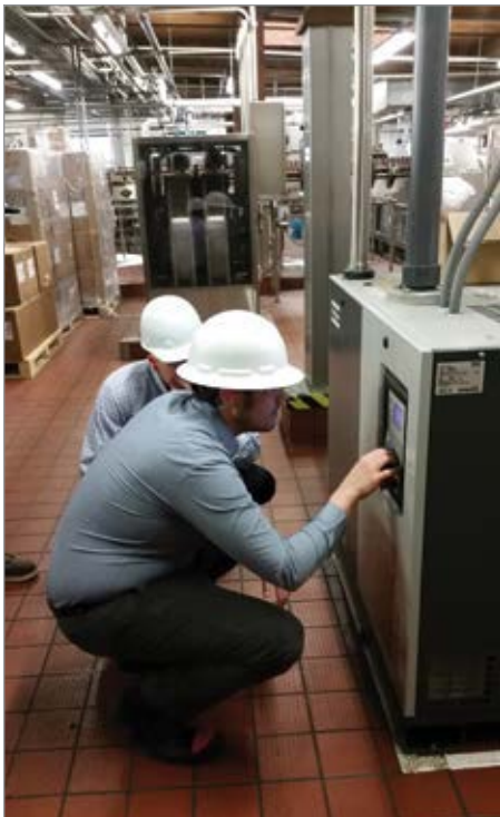
Atlas Copco GHS VSD+ rotary screw vacuum pump at Widmer Brothers Brewery.
