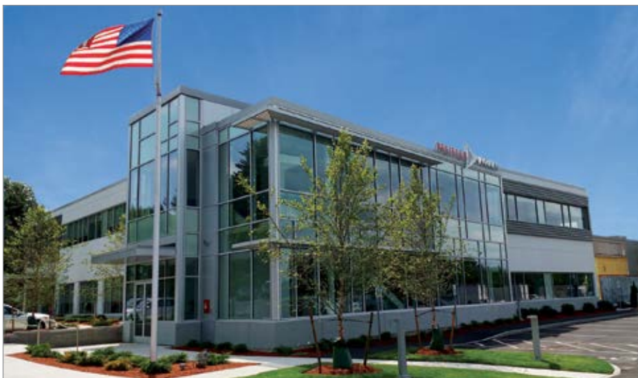
Pfeiffer Vacuum's New North American headquarters facility.
