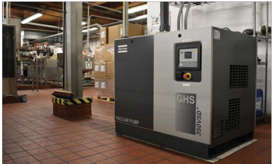
An Atlas Copco GHS VSD+ rotary screw vacuum pump is the first known waterless pump in the craft brewing industry.
