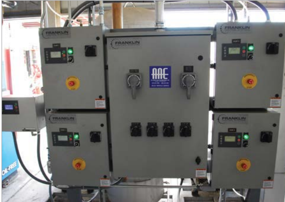
EnerAir's Metacentre V4 master controller fully integrates vacuum equipment for better overall system management.
