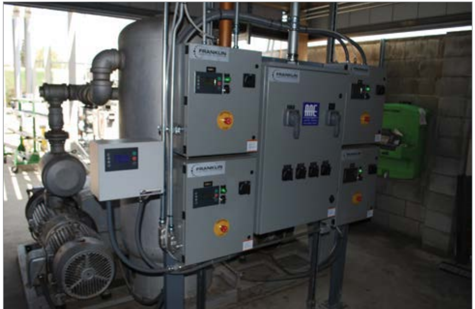
The advanced, yet user-friendly controls of Airmaster help optimize vacuum pump performance.
