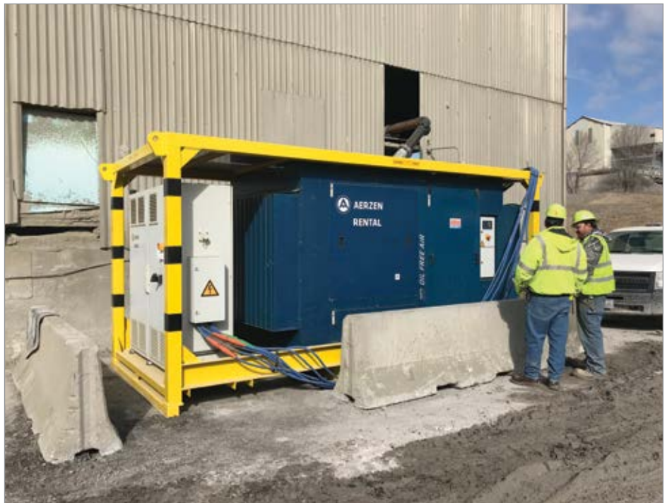
When an air compressor airend failed, a cement company didn't miss a beat by renting a single-stage, oil-free rotary screw air compressor.
