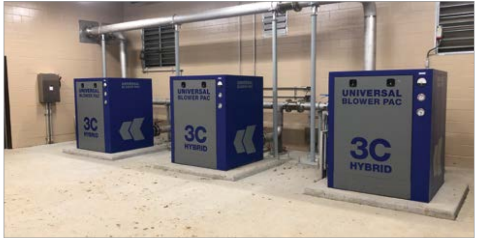
EnviroMix's modified approach to aerobic digestion can use hybrid rotary screw blowers to provide efficient aeration, in turn, satisfying oxygen demand for VS destruction.
