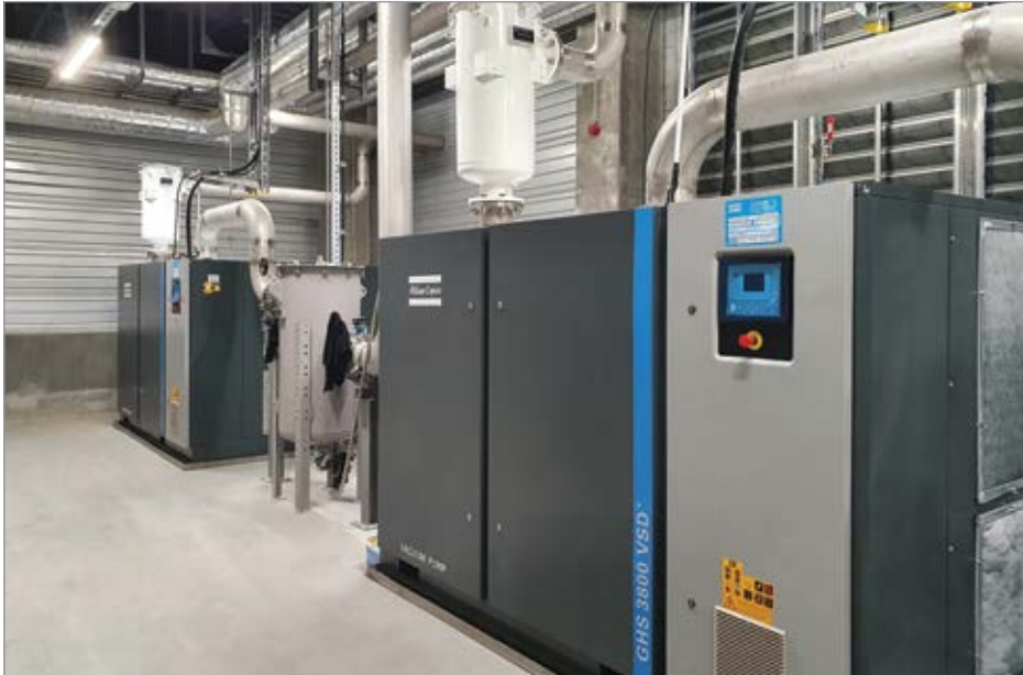
Installation of oil-sealed rotary screw vacuum pumps ideal for a range of applications in plastics, glass, bottling, canning, wood, packaging, printing and paper, meat packaging and many more.
