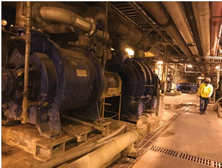
Two of twelve medium-sized liquid ring vacuum pumps on a fine paper machine.
