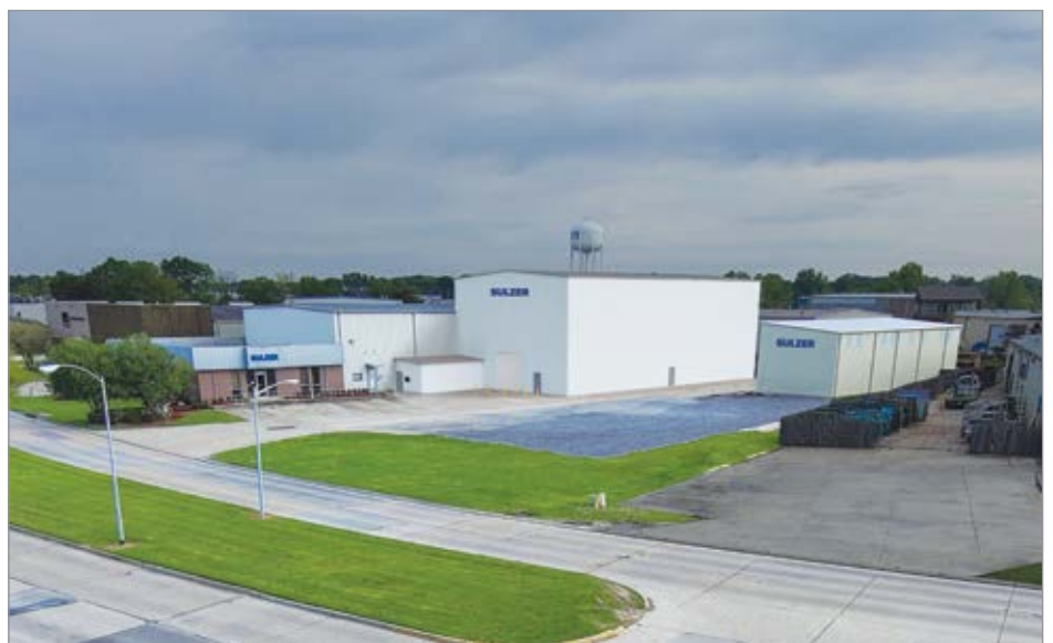
The expansion of the Baton Rouge Service Center will enhance the service capabilities and support for operators of rotating equipment in the US Gulf Coast area.
