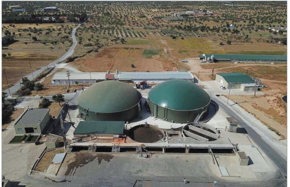
WELTEC expanded this biogas plant the has doubled output by one megawatt.
