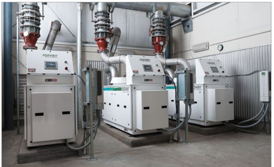
Integrally geared Inovair IM-20 blowers help the plant save energy, while also solving heat and noise issues.
