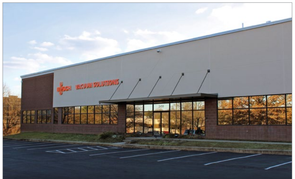
Busch Vacuum Solutions USA new 19,000 square foot Service Center located outside Philadelphia, Pennsylvania USA.
