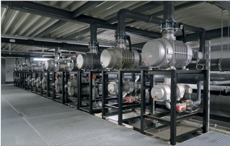
A modular centralized vacuum system solution makes it possible to generate significant savings when it comes to energy and maintenance costs.
